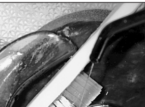
5. Again, as with attachments, clean remaining material with constant use of water, brush and vacuum.
